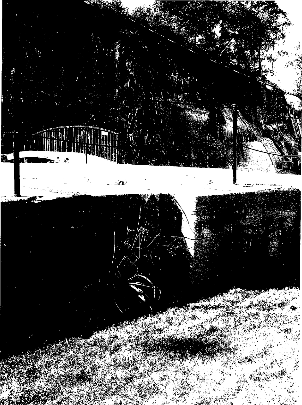
Close up of lower 'door' location.
